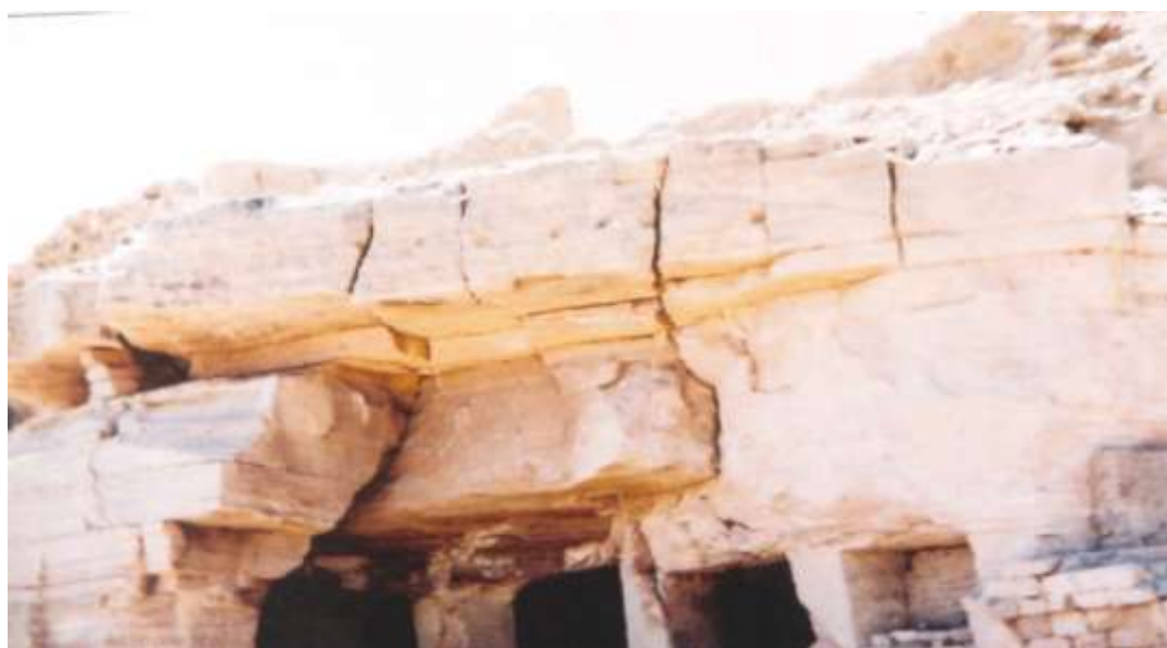
Fig. 4 Details of the serious joints existed in khones tomb.
