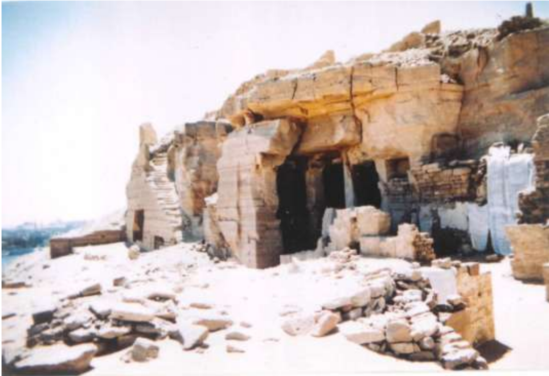
Fig. 1 The joints spreaded in the rock of one of the Elephantine tombs (Khones).
